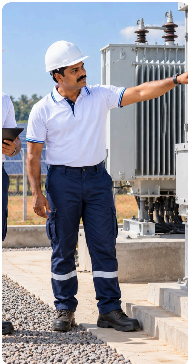
Illustration: inverter station.
