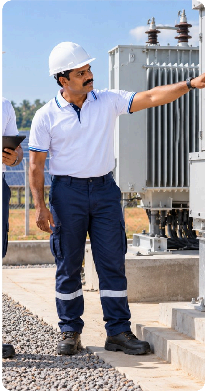
Illustration: inverter station.
